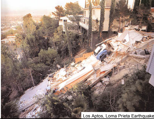
Los Aptos, Loma Prieta Earthquake
